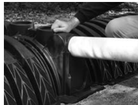
6. Insert connection pipe.
