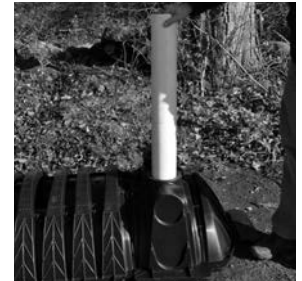
2. Pipe in endcap inspection port.
