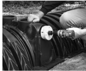
1. Drill endcap on side or top.
